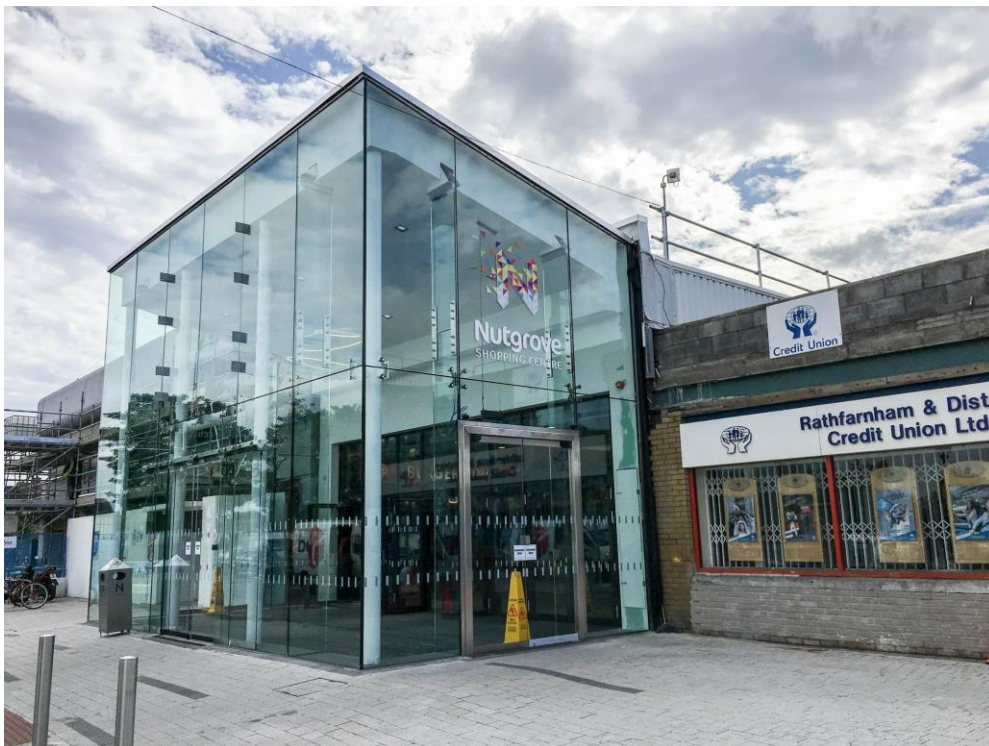
Photo 1: Nutgrove refurbishment work proceeding well
